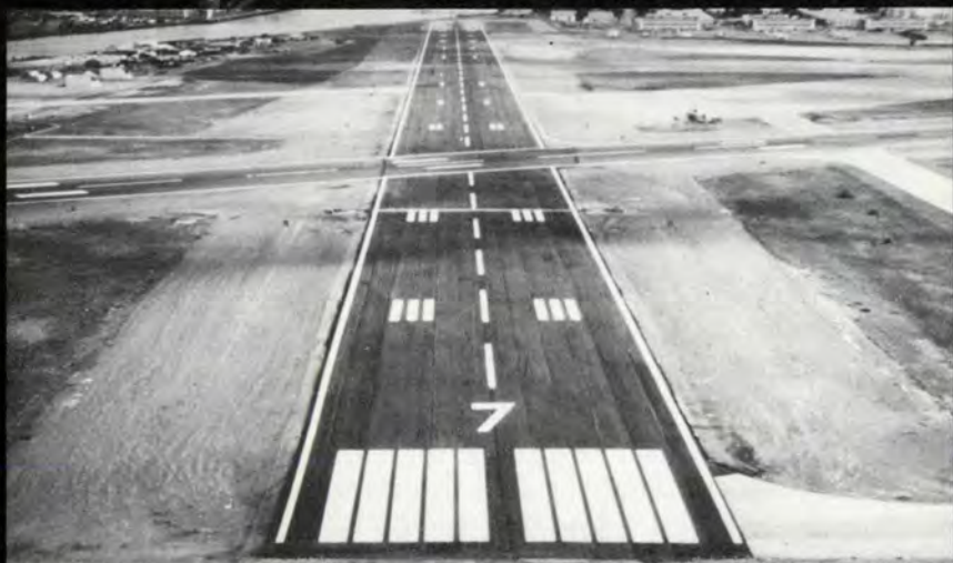
NAS Alameda in San Francisco Bay. Runway 7-25.
